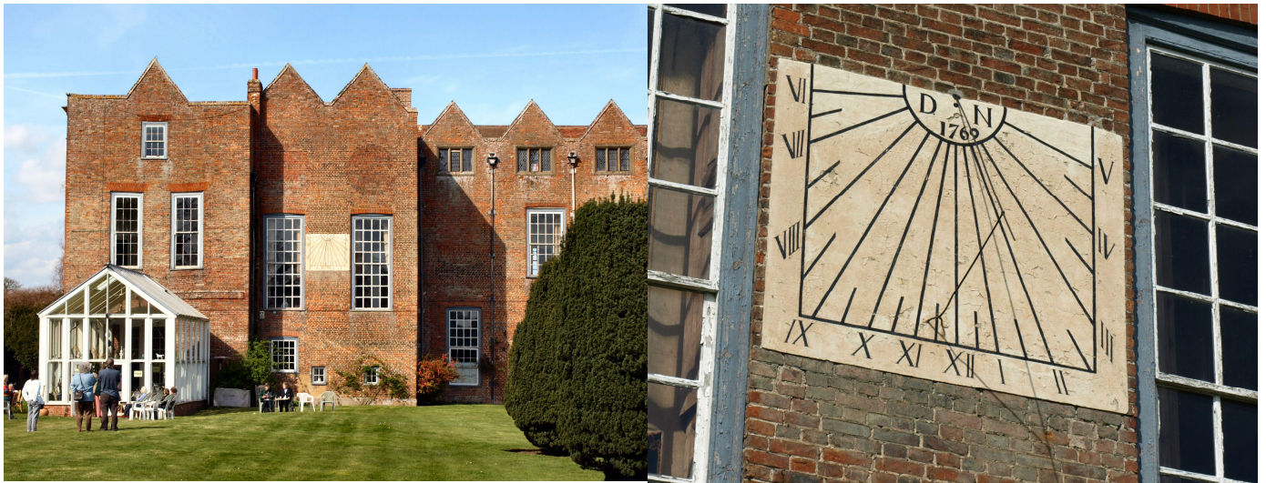
Fig. 2. Left—the south front of Glemham Hall with the vertical dial and mysterious circular marking on the brickwork. Right—close-up of the dial inscribed “D · N 1769”.
